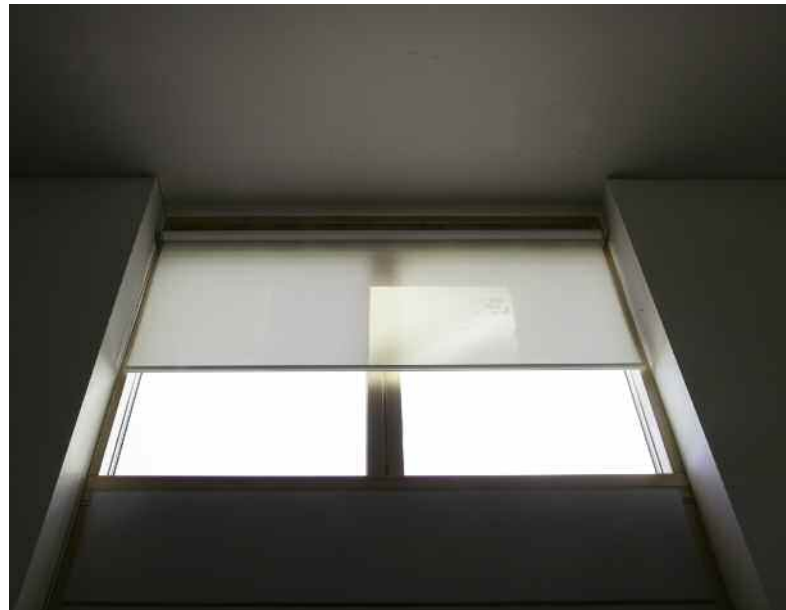
▲ DJA fitted full height, double glazed windows, to give a view of St Paul's Church.
