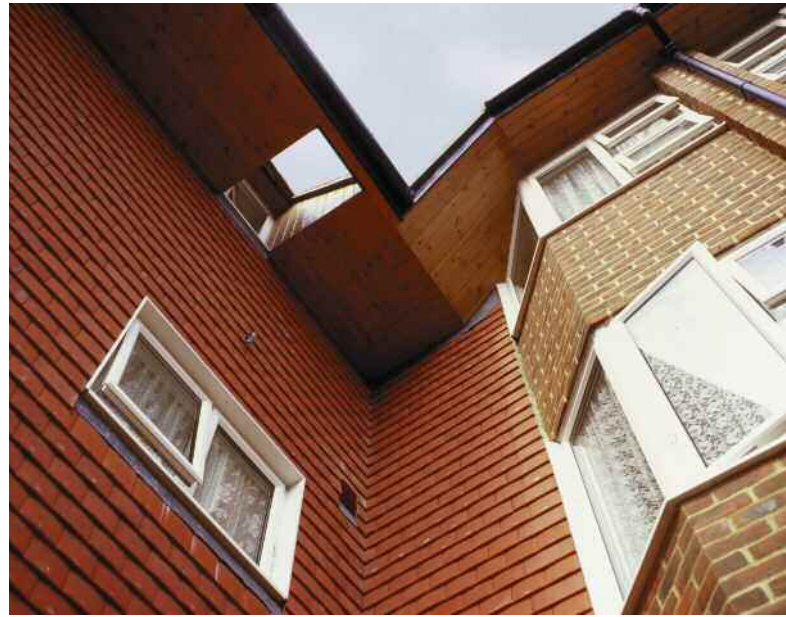
▲ The intricate roof structure, incorporating very wide soffits and large overhanging eaves, contains two third-floor flats within its space.
